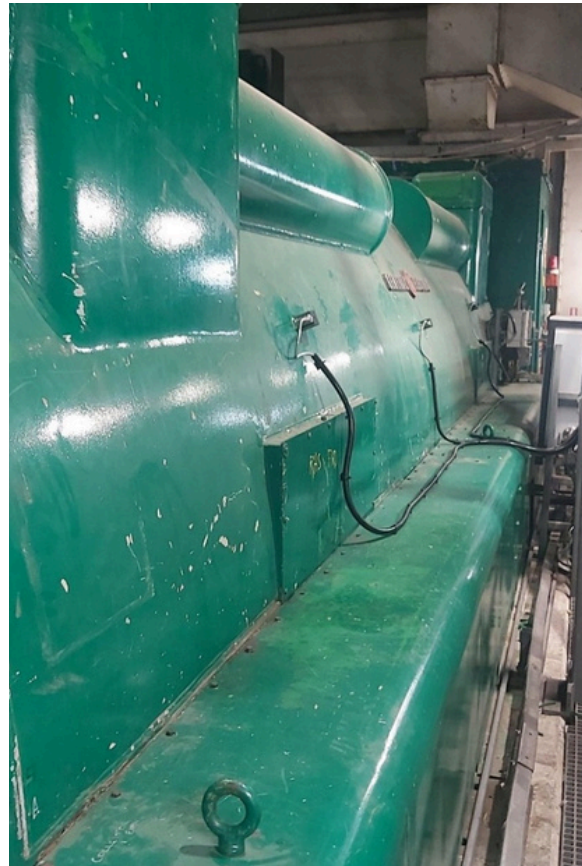
Figure 1: Temporary vibration sensors attached to the generator casing.
