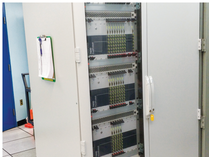
Installed Beran PlantProtech PCMS System configured to monitor NFAC's Fans and Motor Generators.
