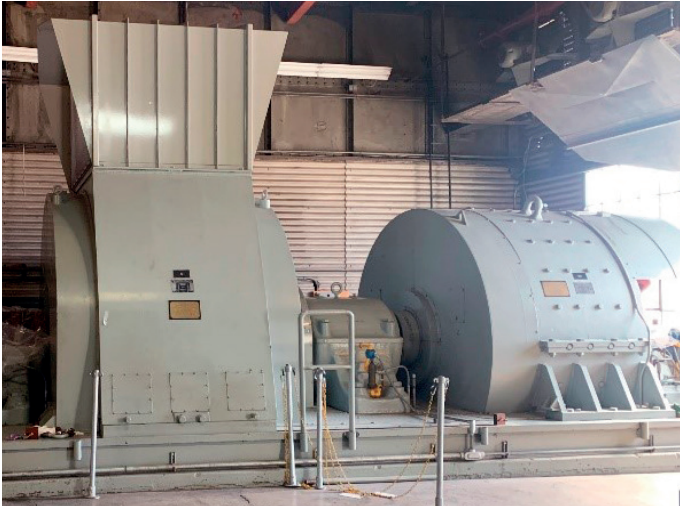
Motor Generator unit in use in the wind tunnel test facility.
