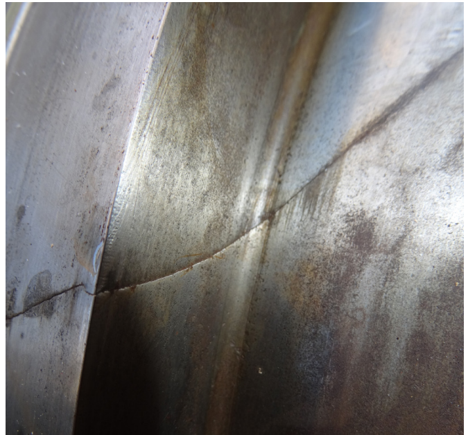
Excessive amplitudes of torsional vibrations can lead to shaft cracking without warning.
